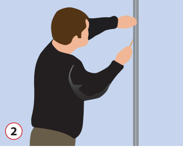
2 Marking out plain walls.
